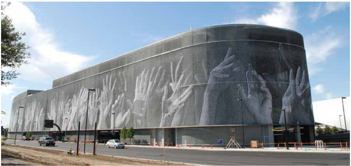
The structure's east façade features dramatic full-length murals that were decided on after the precast had been erected. Embeds in the spandrels allows the artwork to be attached after construction.
