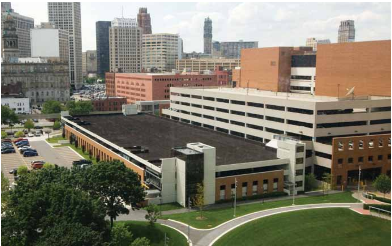
Neumann/Smith Architecture created a plan to remove several levels of a parking structure in Detroit. A 200-kW pv array will be installed on the roof and will generate power equivalent to the annual needs of 40 homes.
