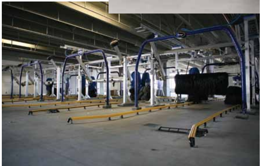
The quick turnaround area features special services for washing (bottom) and refueling (top) vehicles, the first time such activities have been provided on elevated levels of a parking structure.
