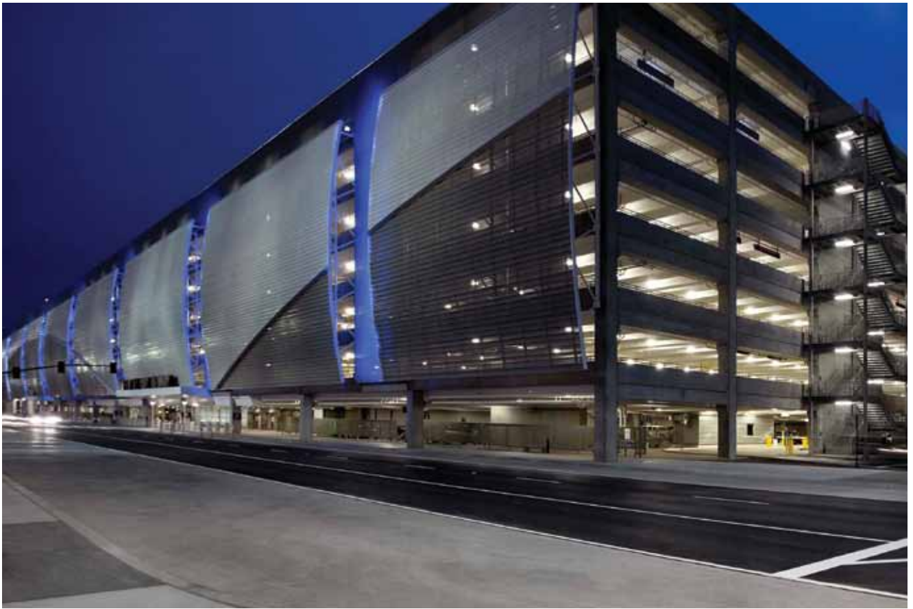
The structure's west façade features architectural metal panels and mesh to dampen lighting and create an attractive finish.
