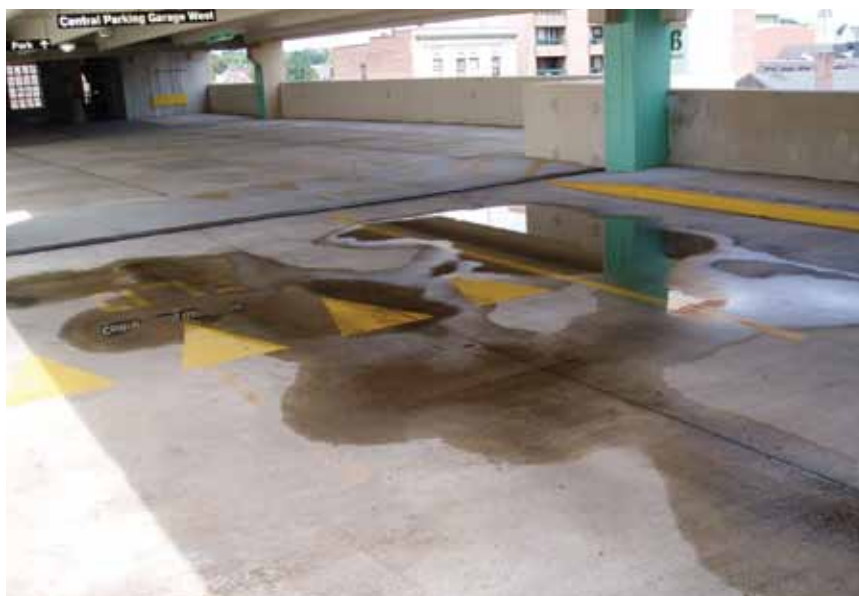
A key goal for designers when planning the structure is to work to eliminate any aspects that encourage water ponding, which can increase water penetration into the concrete and the potential for freeze-thaw damage.
